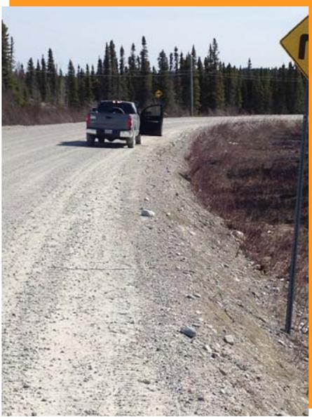
Photo 63: 2+005 à 2+140 – Washouts potential of talus if paving
