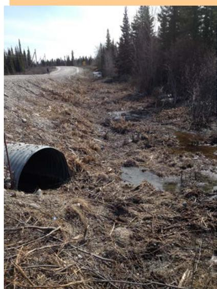
Photo 68: 2+400 TTOG 900 D – Outlet clearing required – Take-off ditches
