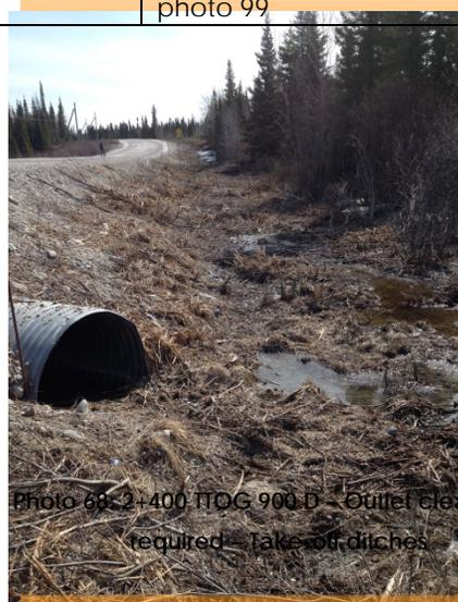
Photo 68: 2+400 TTOG 900 D – Outlet clearing required – Take-off ditches
