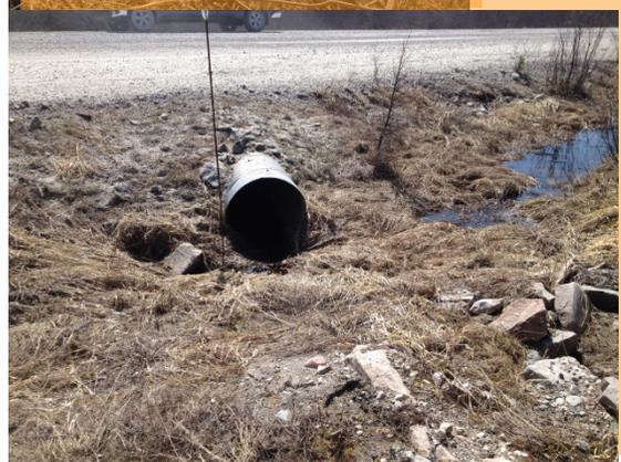
Photo 99: 15+400 TTOG 900 – Inlet clearing required
