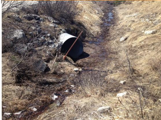
Photo 92: 13+800 TTOG 1200 – Inlet clearing required
