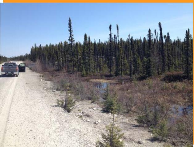
Photo 94: 14+050 à 14+250 – Accumulations of water trapped by terrain (roc)
