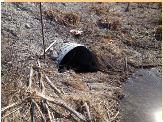
Photo 64: 2+300 TTOG 900 D – Outlet clearing required
