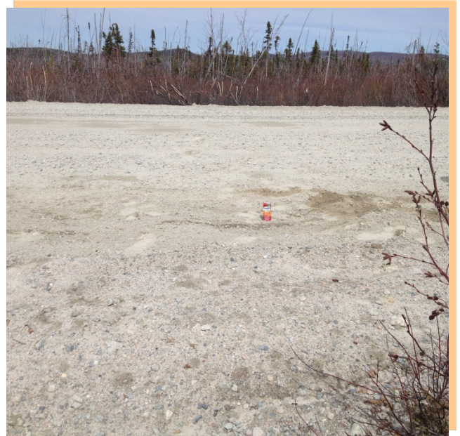
Photo 20: 4+500 Sub-base Course aggregate – Surface
