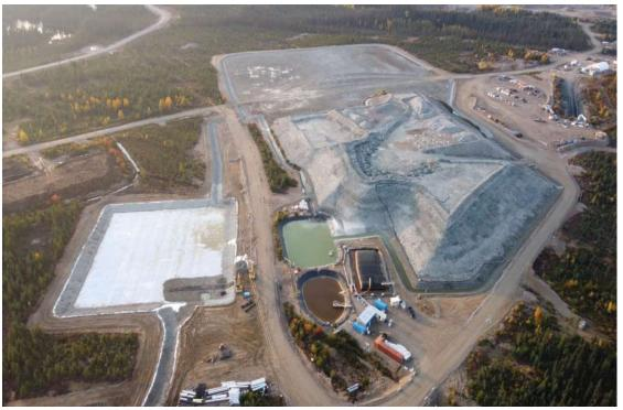
Photo 1: Expansion of the waste rock stockpile and construction of a new pond
