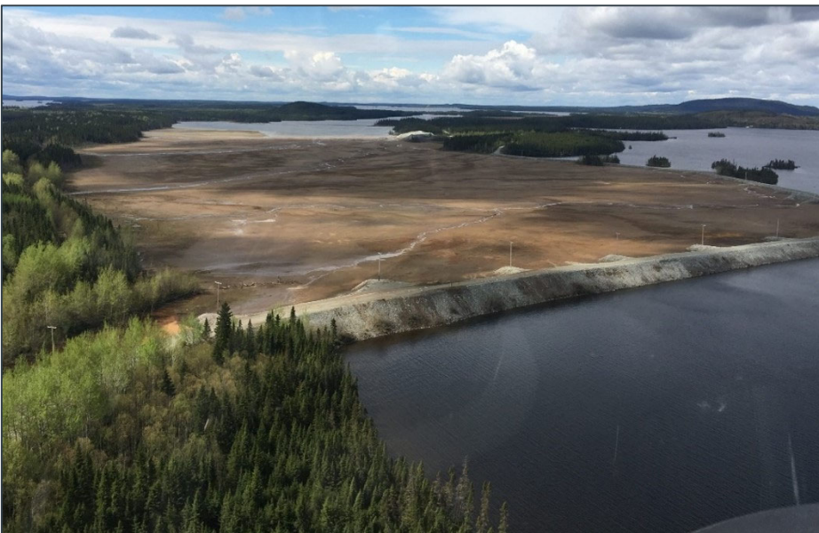
Figure 8: Tailings facility - Copper Rand
