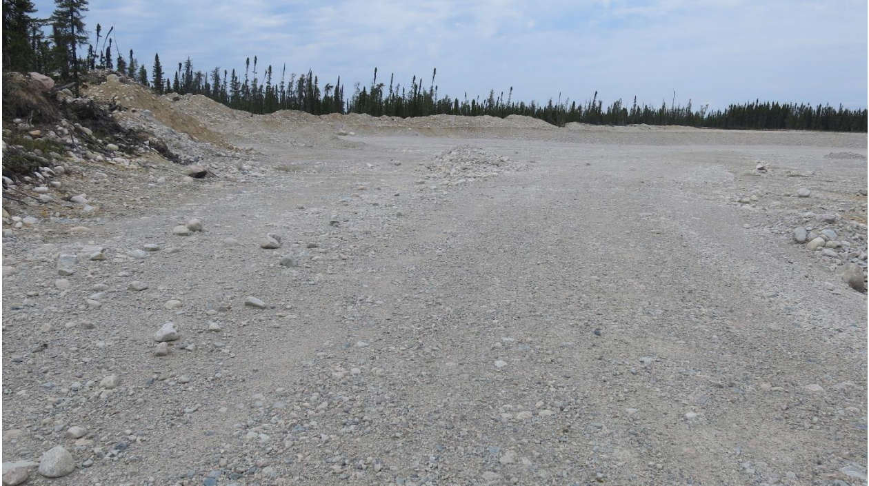
Photo 1 : Central portion of the GD-17 borrow pit.
